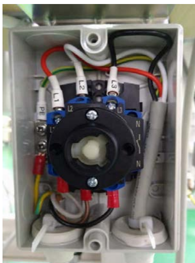
Power supply connection, 3-phase, 200-240 V
